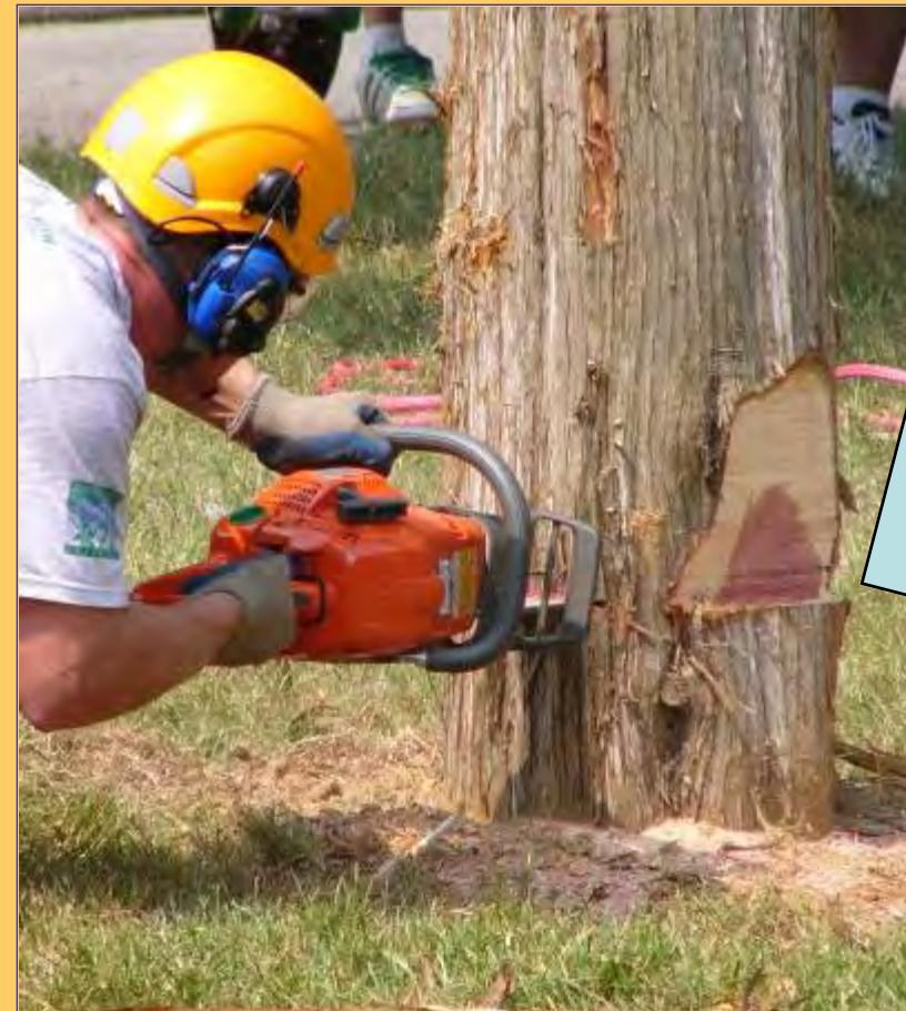
Here a bore cut is used to form the back cut. Note that it is level with the apex of the notch.
